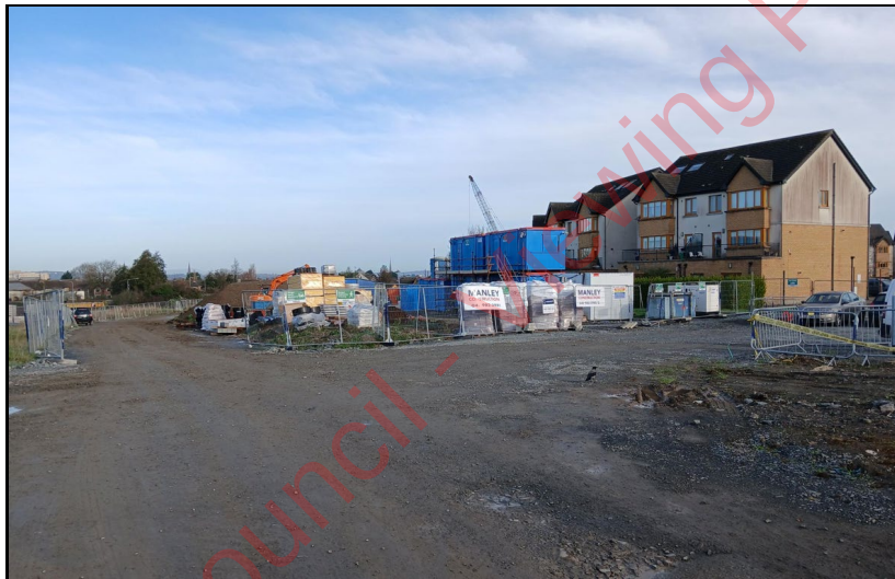
View of application site looking northeast
