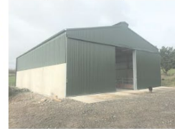
Picture 2 Example of Typical modern farm building
