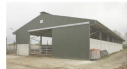
Picture 1 Example of Typical modern farm building
